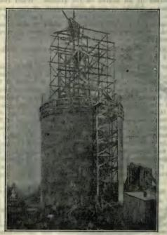
Fig. 23.—Erecting Concrete Standpipe.
